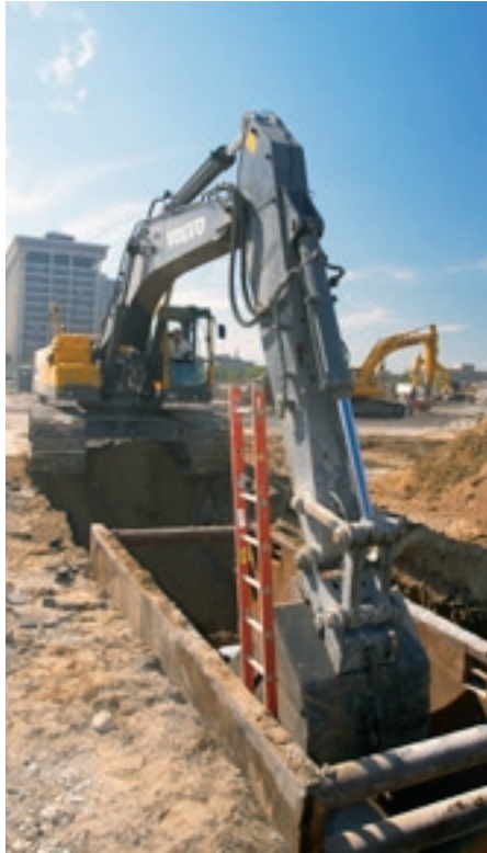
Utilities excavation kept things moving.
