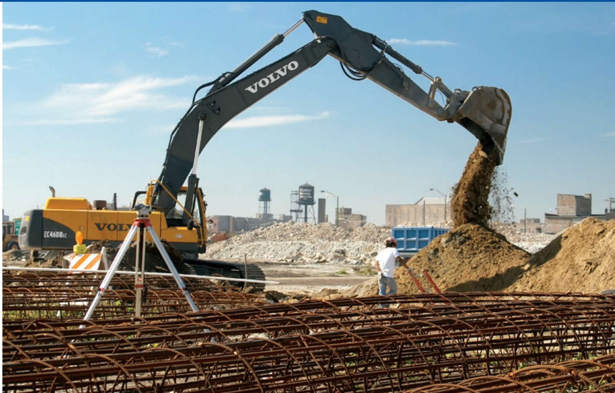
The massive 27-acre expansion of McCormick Place posed significant challenges
