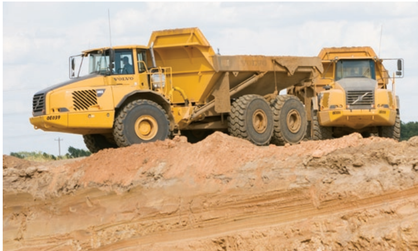
Volvo A40D artics haul sand at the LMC sand mine in Ambrose, Texas. At Right: working sand and stone at a rail facility.
